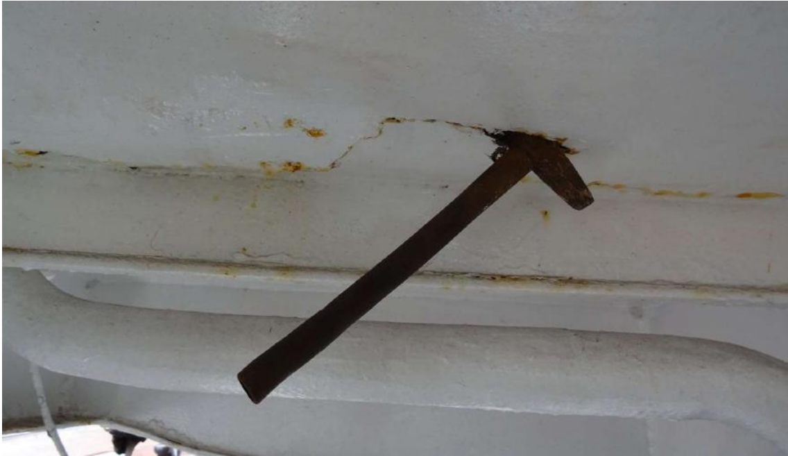
Fig. 5. 3. Testing integrity of the steel by chipping. Source: Deutsche Flagge.
