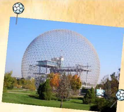
The geodesic dome as designed by Richard Buckminster Fuller for the 1967 Montreal EXPO.
