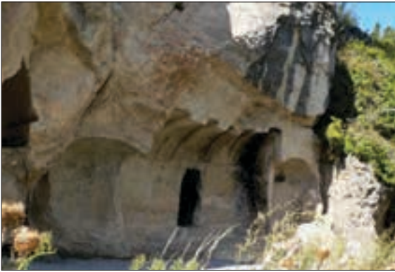
Figure 1.9 Las Gobas 4–6 (Laño, Treviño County, Burgos), a complex of caves carved in a Danian-aged dolostone unit, circa VII century (above); ruins of a worship cave (left). Photographs looking north.
