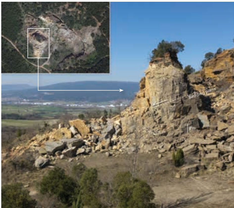
Figure 5.4 Significant rock falls from ‘the pinnacle’ of Gometxa quarry, which occurred at the end of 2013. The pinnacle is about 18 m high and was left by the quarrying operations, note the strata dip running into quarry. Photograph taken on 7 March 2014, view to the northwest. The inset is an aerial orthophoto of the quarry taken in 2015, spatial resolution of 0.25 m (source: GeoEuskadi, www.geo.euskadi.net ).
