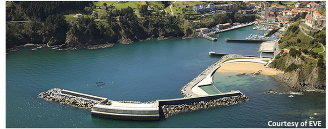
Fig. 2. Aerial view of the Mutriku Wave power plant.
