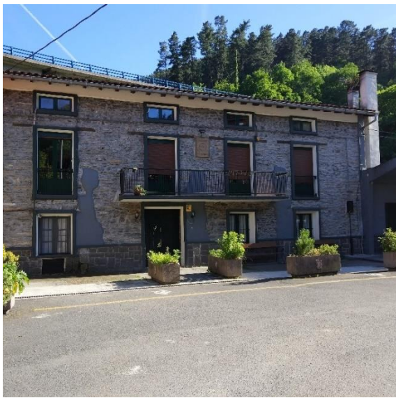
Fachada principal (Norte)
