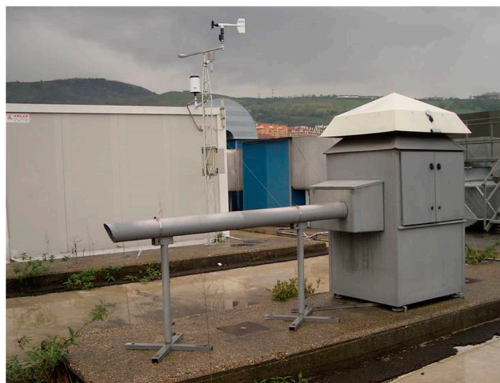
Figure 2. Photography of the sampling place on the roof of the Faculty of Engineering.
