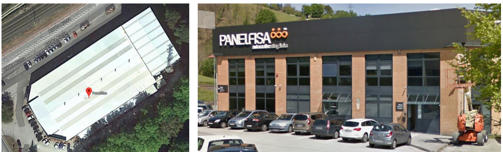
Fig. 1. Aerial view of the building, highlighting the administrative area (left) and view of the exterior facade of the administrative area (right). Source: Google Maps.
