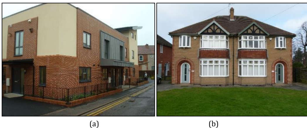
Figure 35. (a) North side of Gainsborough house [99] (b) Front side of Loughborough house [100].
