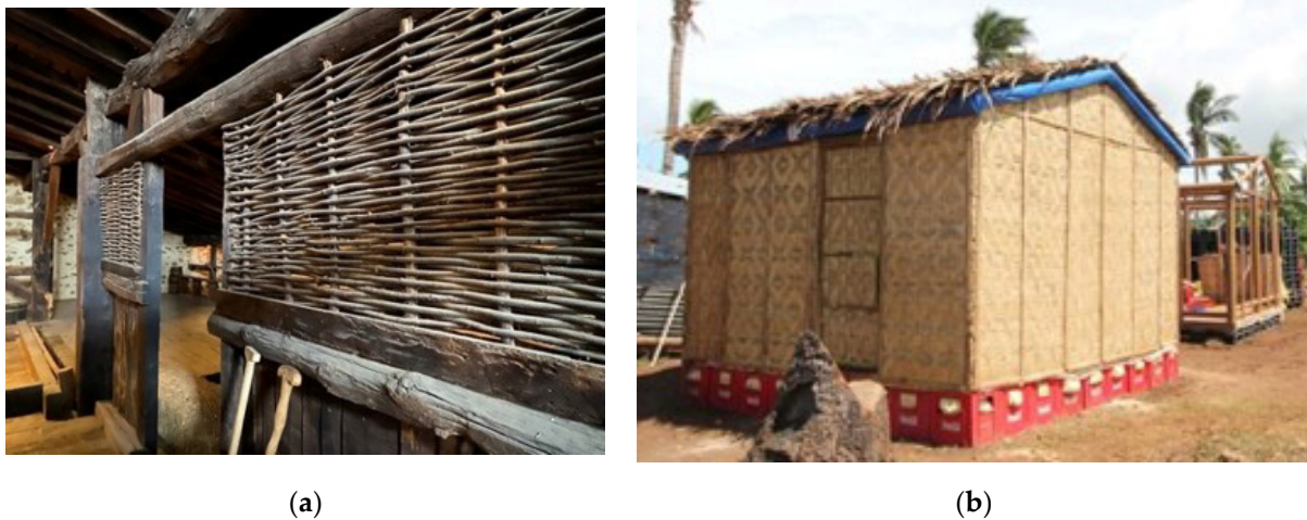
Figure 1. (a) Interior partition of the Basque farmhouse “Igartubeiti” made with basketry techniques [7]; (b) Temporary shelters in Cebu, Philippines [8].
