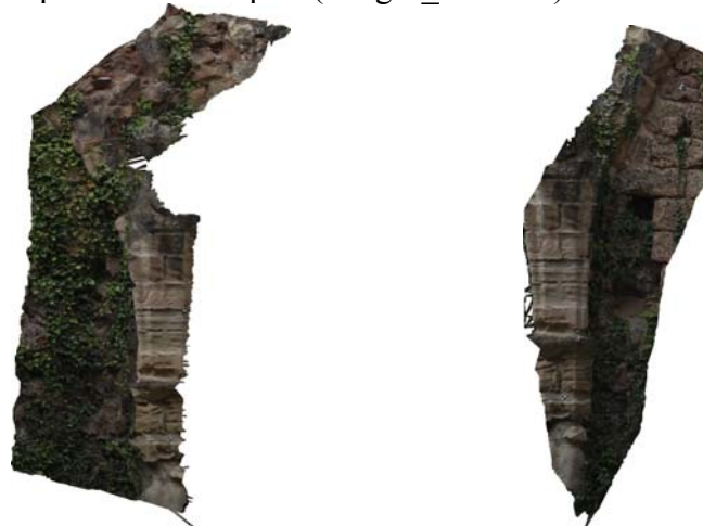
Images_55 & 56 : Orthophotos of the column (southern wall)
