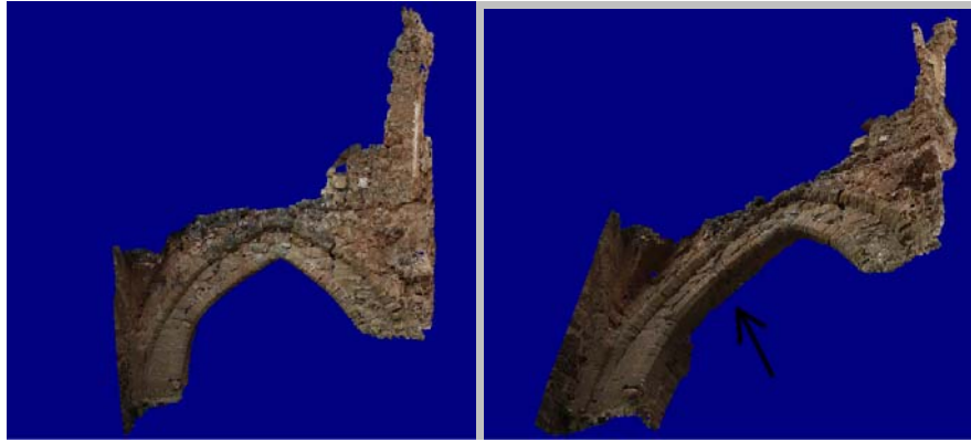
Images_44: The western wall
