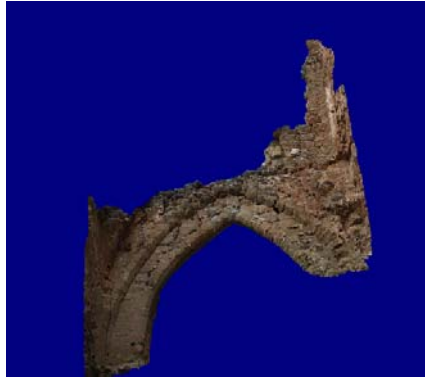
Image_73: Point Cloud of western wall
