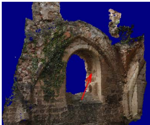
Image_41: Point cloud of the western part of the southern wall created all in one project (one orientation)
