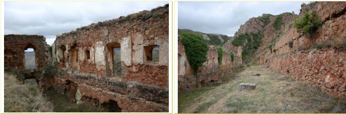
F.- Big building in “L”, inside.
